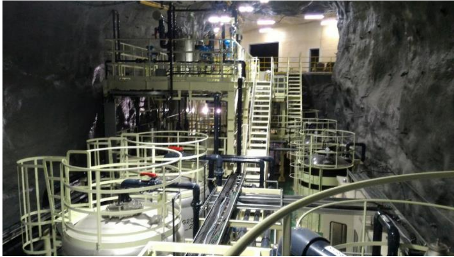
Gd-loading, pre-cleaning and Gd-water circulation systems were constructed.
