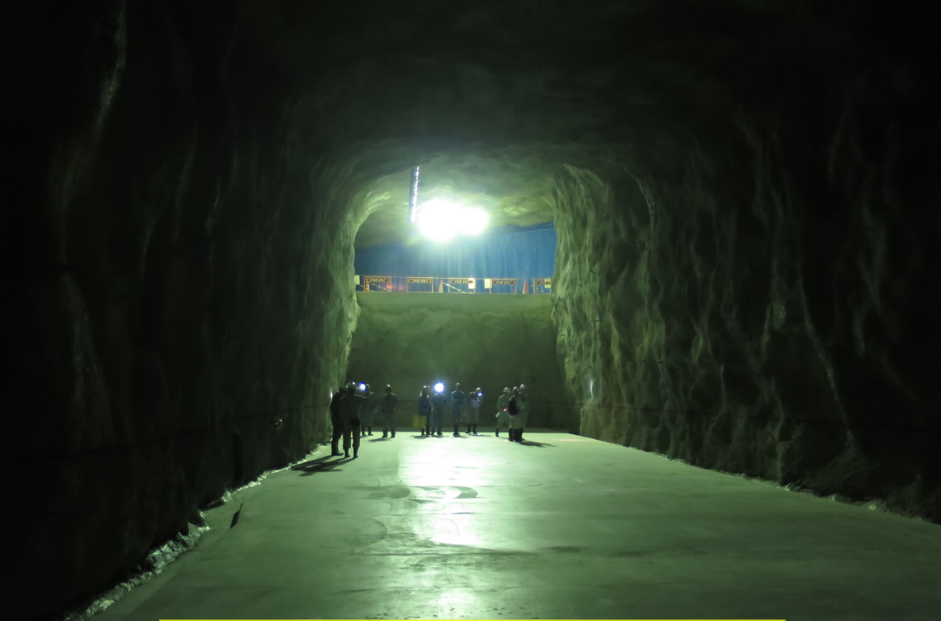
New gadolinium water system hall (“Hall G”); September 10 st , 2015
