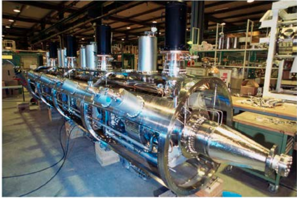
Main 400MHz RF Accelerating System Accelerating System (Four-Cavity Cryomodule)
