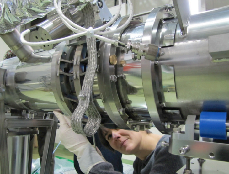
Serena Barbanotti from FNAL installed magnetic shield
