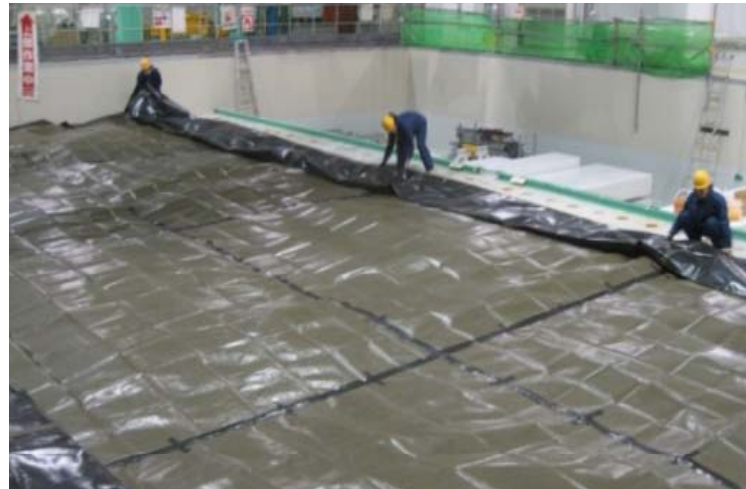
Lay the protection sheet under air-tight sheet
