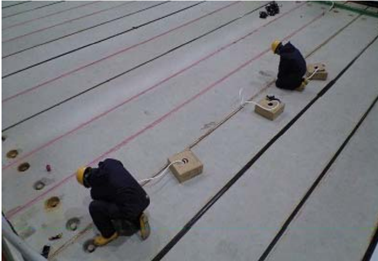
Caulking between concrete shields
