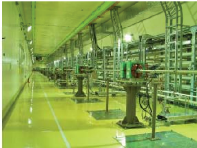
ACS modules were installed in the tunnel
