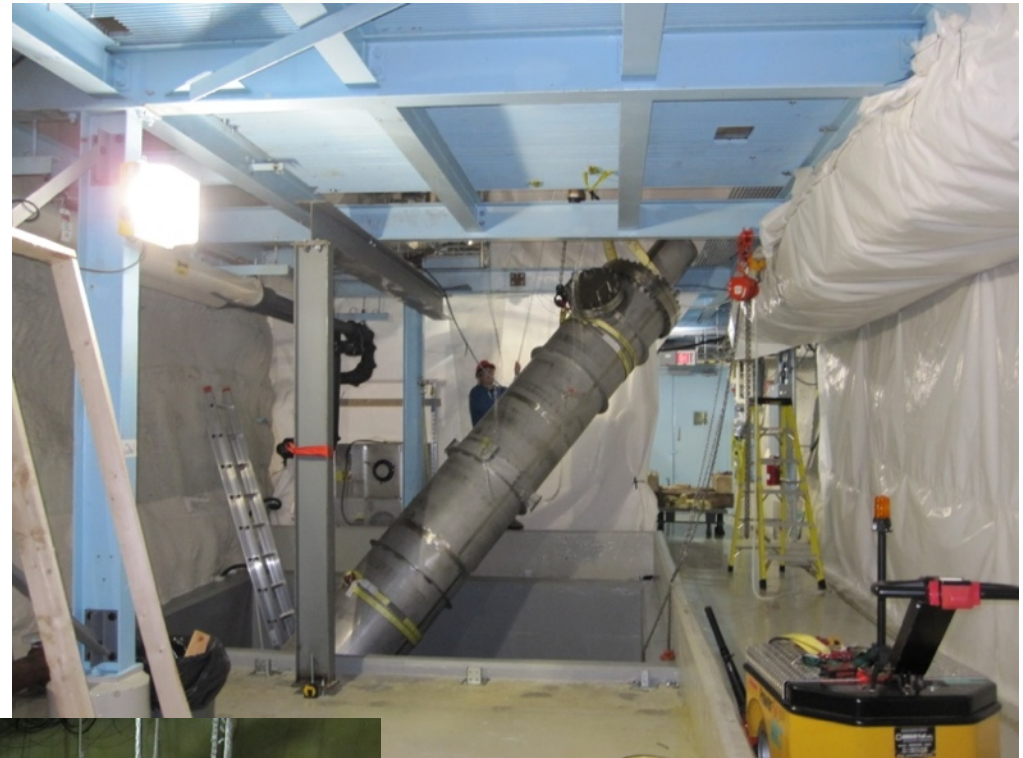
First LAB plant vessel being installed into utility drift (prior to completion of steelwork)
