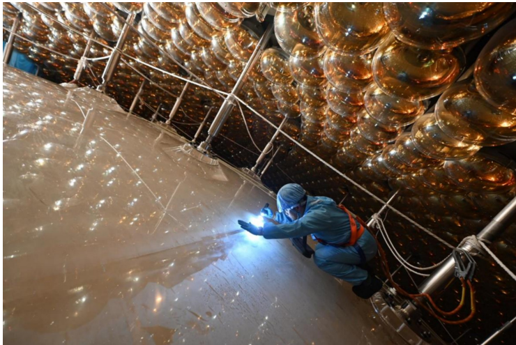
Inspection of bonding lines.
