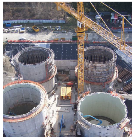
Waste-water treatment facility (~30m water depth)
